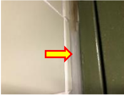
Photo 9: Pipe Chase Door in Men's Washroom.
