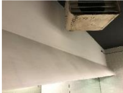
Photo 6: Bulkhead above sinks – Women's Washroom.
