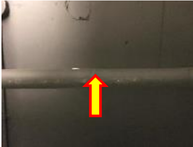
Photo 3: Non-asbestos pipe insulation – Men's Washroom.
