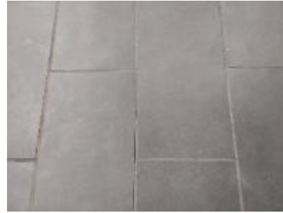
Photo 11: Ceramic floor tiles – Women’s Washroom.
