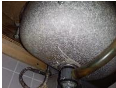
Photo 12: Undercoating on sink – Women’s Washroom.
