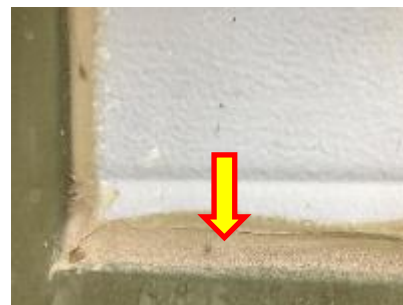
Photo 8: Exterior Door of Men's Washroom.
