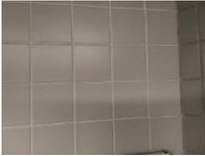
Photo 10: Ceramic wall tiles – Women’s Washroom.
