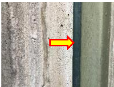
Photo 7: Exterior Door of Women's Washroom.
